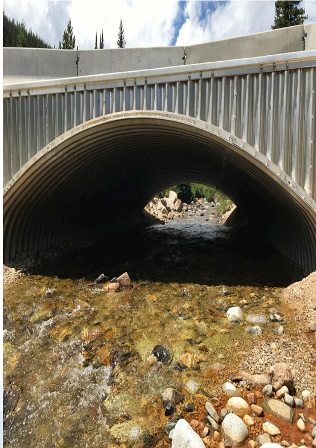
Bottomless culvert above Turquoise Lake Photo: JW Associates Brad Piehl
